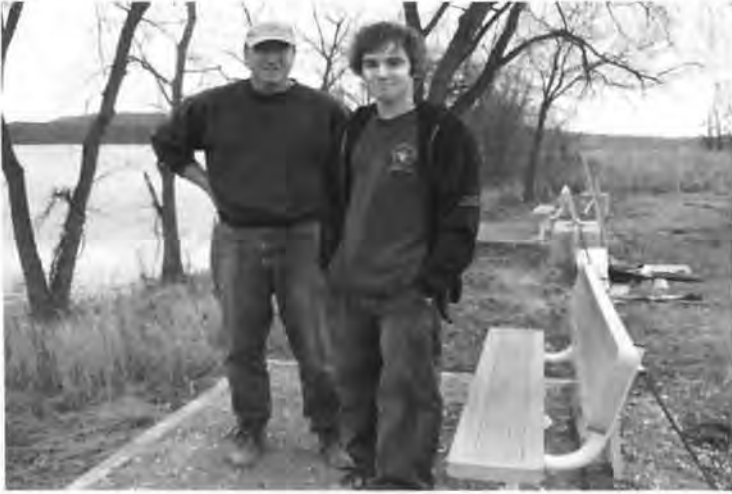
Jeff Rowe (left, proud father) and Allen Rowe take a moment to pause beside the steel benches they are constructing overlooking Oxbow Lake. As his Eagle Scout project, Allen Rowe planned, organized, and obtained funding from Indiana Michigan Power for a clean-up of the entrance parking area and the installation of the benches at the Oxbow Lake Overlook parking area. (photo by Jon Seymour)
