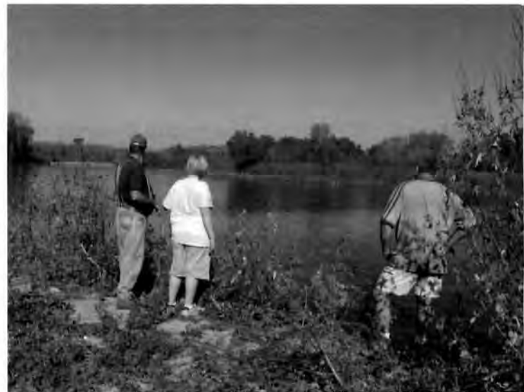
(left to right) Stanley Craig, area farmer, Kaleb Gillespie, Stanley's grandson, and Bob Minges, FOGM, inspect the eroding west bank of the Great Miami River just above the railroad bridge. Friends of the Great Miami started a reforestation project along a 1/3 mile stretch of the river bank, on Oxbow property, to stabilize the river bank. (photo by Jon Seymour)
