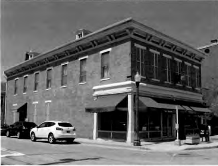
Oxbow, Inc. has rented the corner office at 301 Walnut St. as their first ever home. The storefront will serve as the office and storage area in the rear and a combination of meeting space and educational area in the front. The location in an historic building, owned by the Knights of Columbus, in the center of Downtown Lawrenceburg was made possible in part by a grant from the Earl and Florence Simmonds Foundation. (photo by Jon Seymour)
