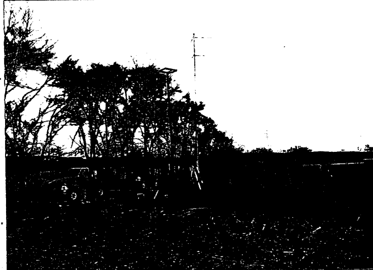
The final height of the telescoping tower is achieved at 30 ft. in the air. (photo by Jon Seymour)
