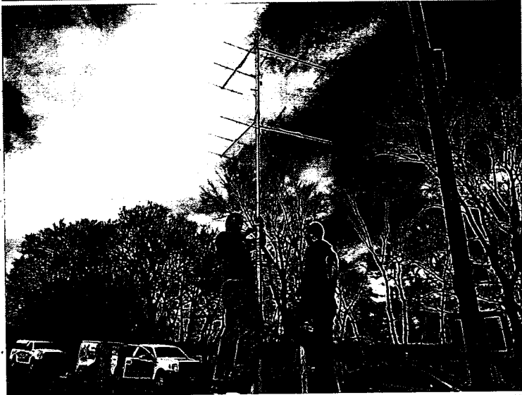
Matt Strauseberg (L) and Sean Langley install the telemetry tower and prepare to hoist it to its operating height. Dr. Krauel offers encouragement and a practiced eye for leveling. (photo by Jon Seymour)
